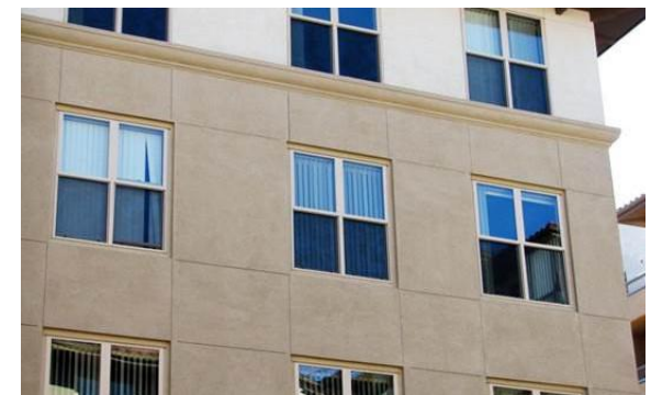
Figure 5.3 Example Expansion Joint Alignment
