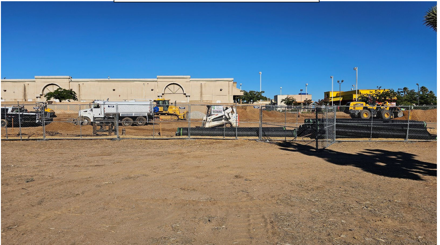
CENTER OF SITE LOOKING WEST
