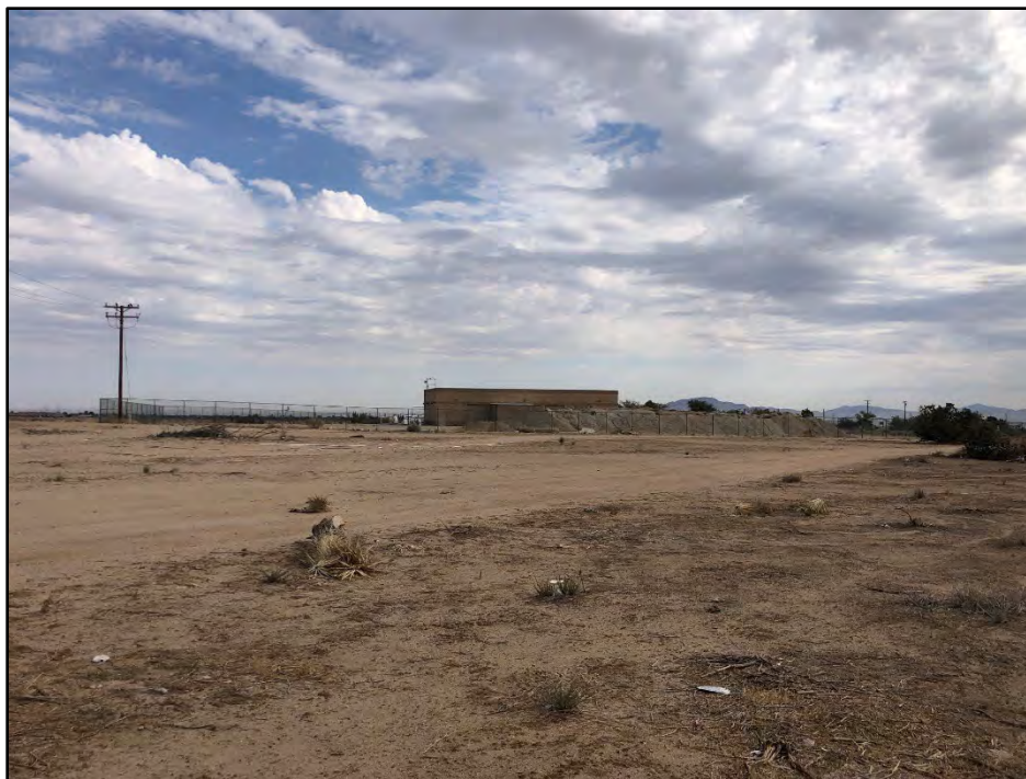
Building located on the Project area. View to north.
