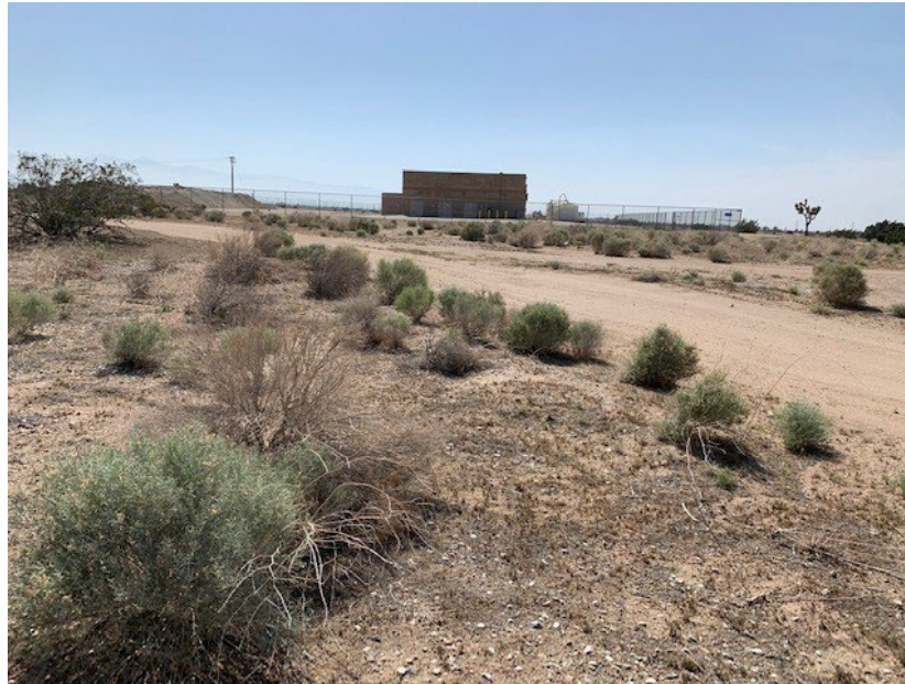
Photograph 3. Looking Northwest at adjacent off-site utilities.
