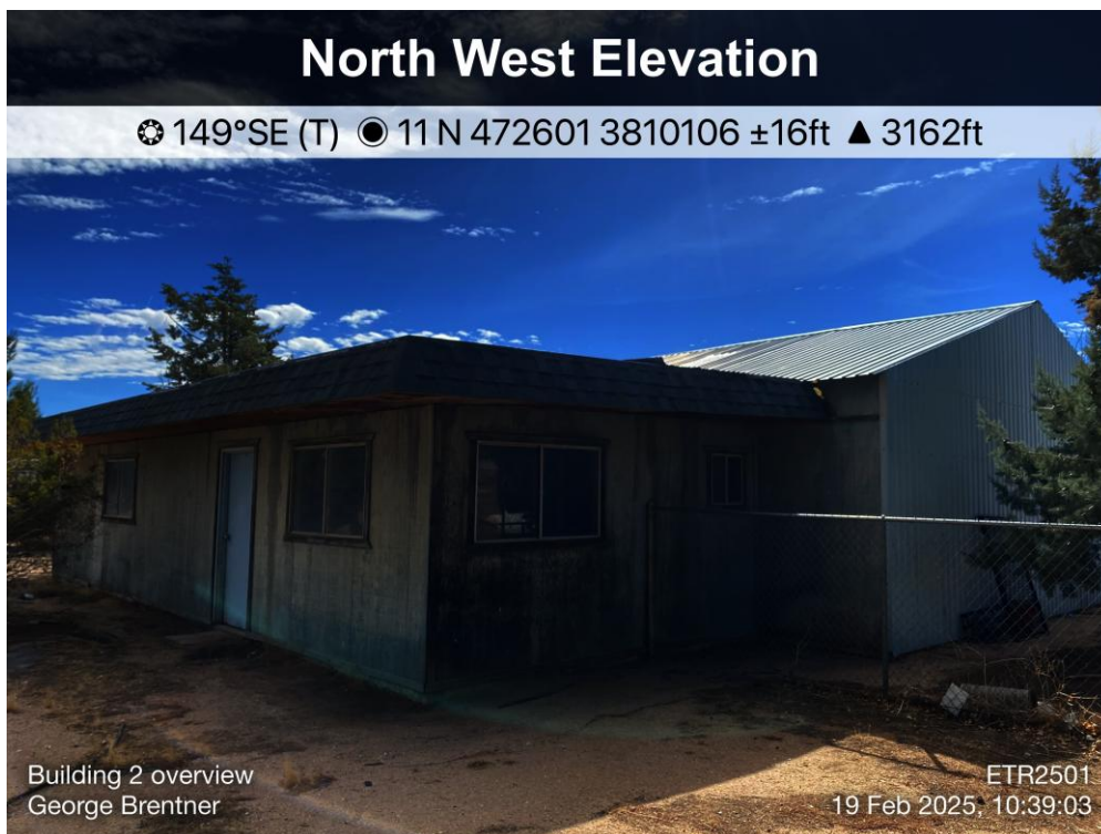
Photo 6: Overview of ETR2501-H-2
