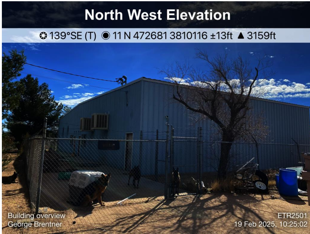
Photo 5: Overview of ETR2501-H-1
