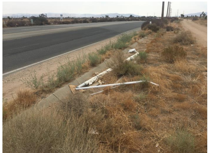
View of concrete drainage ditch along northern property boundary
