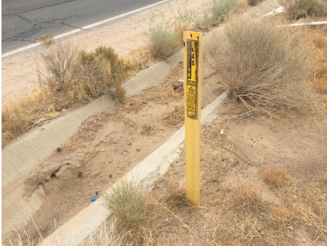
View of natural gas pipeline signage along northern property boundary
